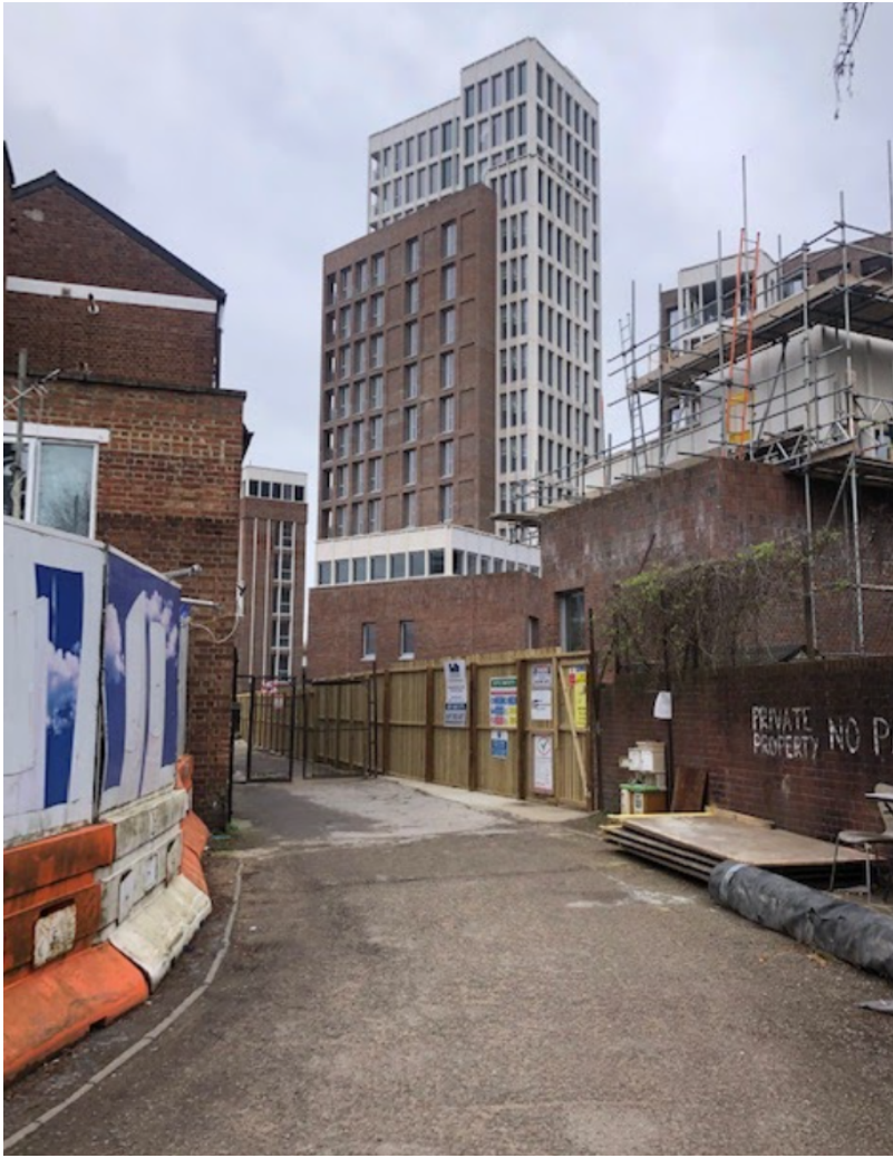
Site with new development to rear
